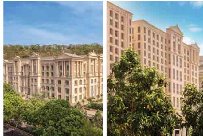
DOWNTOWN POWAI - COMMERCIAL/IT PARK, MUMBAI
