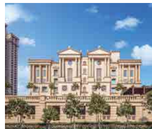
Downtown Powai - Commercial/IT Park, Mumbai
